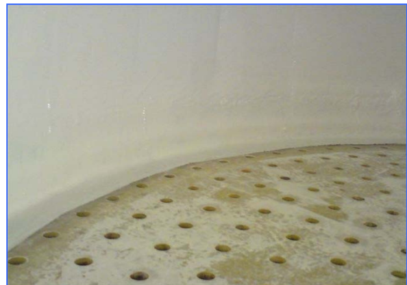
Finishing coat of the inner surface of the filter
