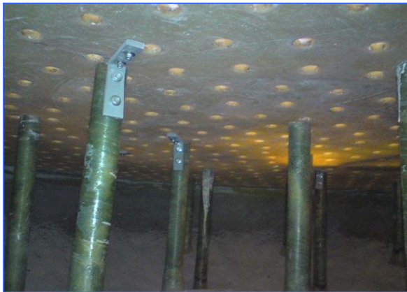
Reinforcement of the filter floor on rear side
