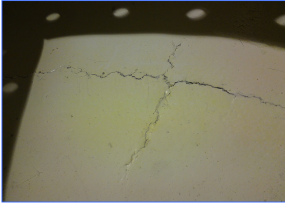
Cross draft of a composite filter floor
