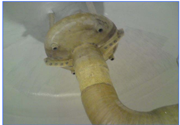
Application of inner surface of delivery pipe
