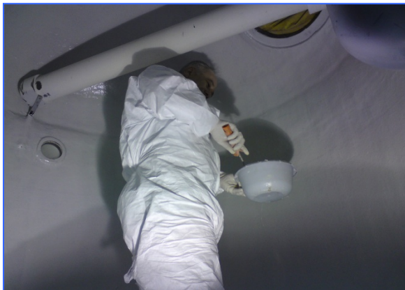
Coating of the cleansing filter
